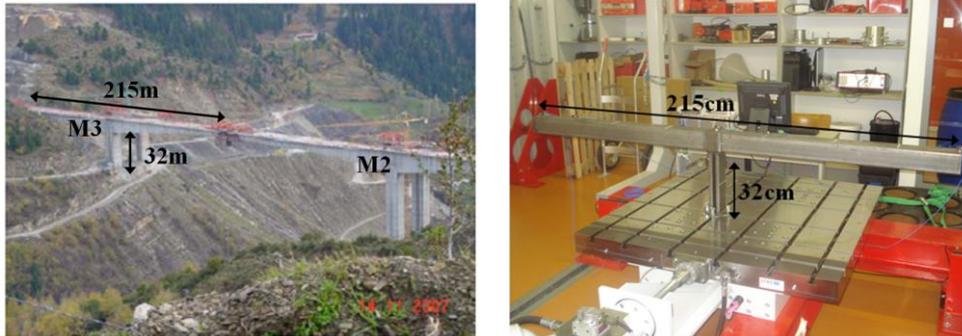
Figure 1. Metsovo Bridge segments under during the construction stage (left) and its equivalent scaled structure tested at the laboratory (right).
